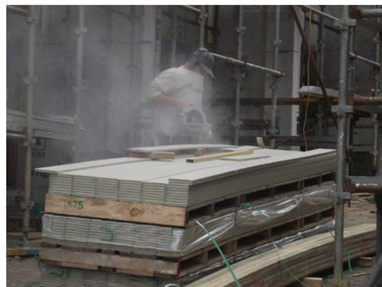
Dust exposure while working with fibre cement products.
